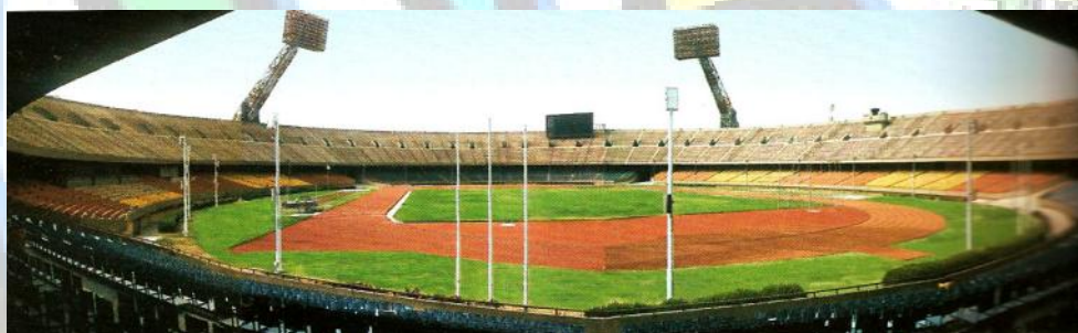
I.G. Stadium Sports Complex
